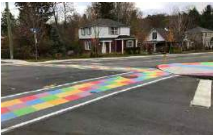
FIGURE 92 - Traverses piétonnes distinctives, Granby © Provencher_Roy
